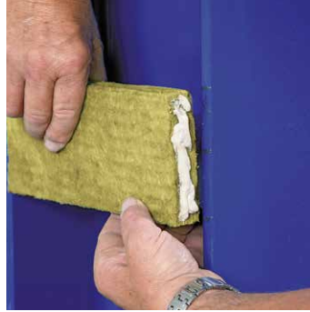
Pose des supports
